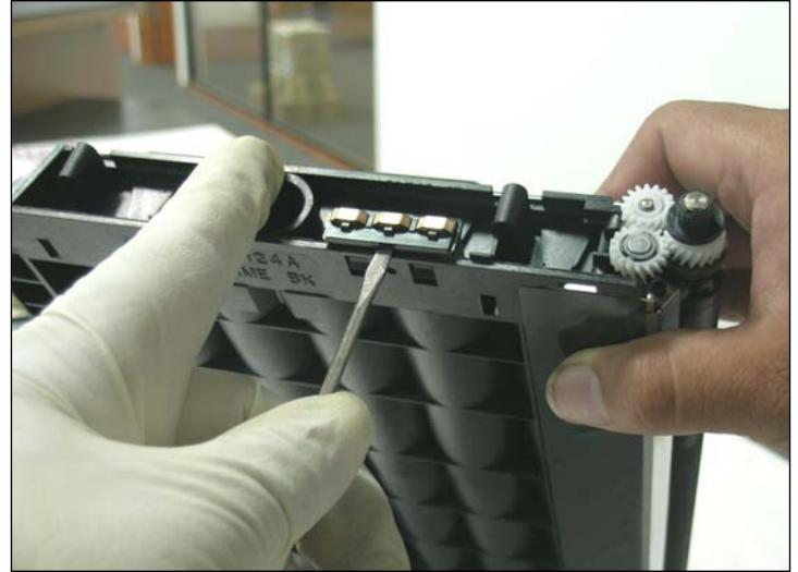
**3. Using a small flat-head screwdriver, carefully pry loose the cartridge contacts assembly located near the toner fill plug on the side of the cartridge.**
